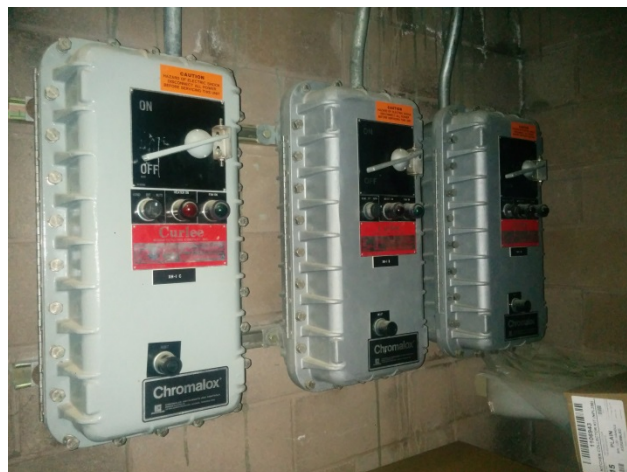
Explosion Proof Control Switches, typical in H-2 occupancies
